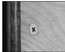
Plywood to steel or wood studs.
