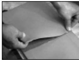
2. Position second Dekstrip over tape & press in place.
