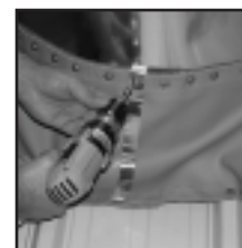
5. Fasten through top of termination strip, Dekstrip, and back of strip with Scots® fasteners or rivets.
