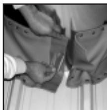
2. Remove film from top of splice tape.
